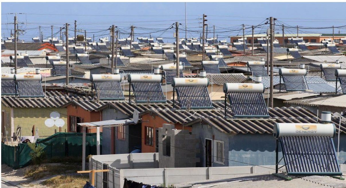
Figure 4-2: Use of solar energy in South Africa townships
